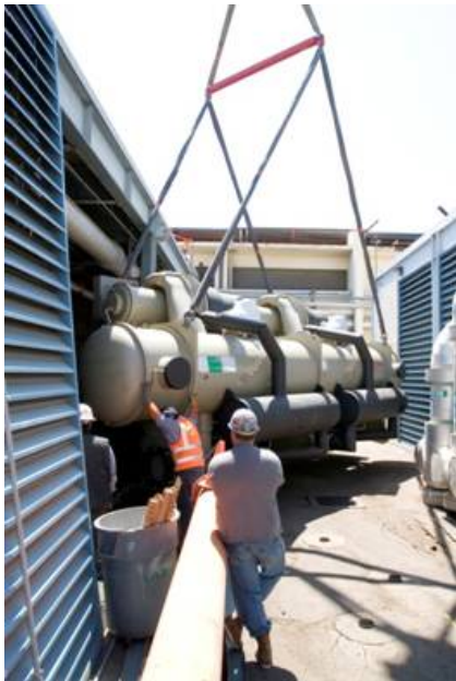
Installation of High-Efficiency Chiller
