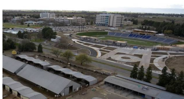
Dairy and Stadium
